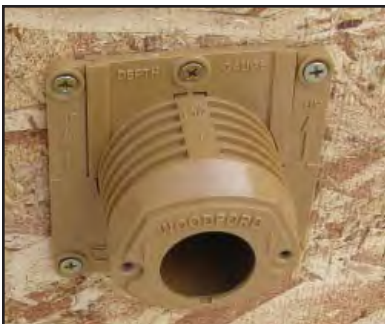
Mounting Sleeve adjusted for depth and attached to wall
